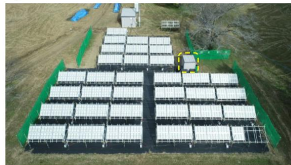
100m 2 SrTiO 3 'photocatalyst sheet' demonstration plant
