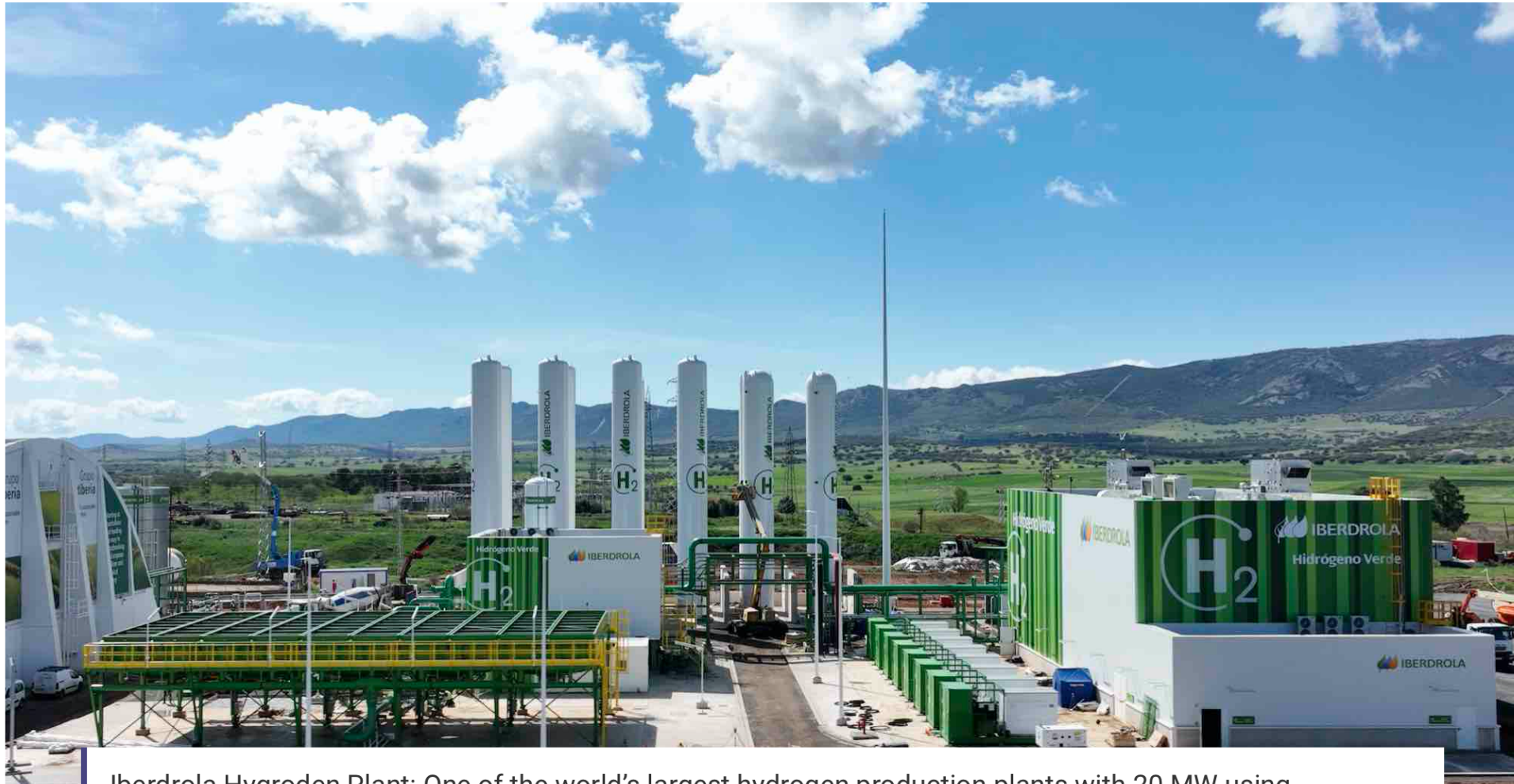
Iberdrola Hydrogen Plant: One of the world's largest hydrogen production plants with 20 MW using electrolysis powered by 100% renewable sources (Image: © Iberdrola)
