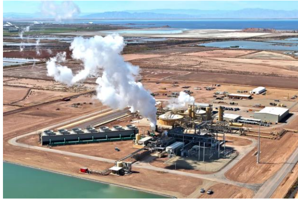
CTR plant, Salton Sea (USA) $520M 50 MW, 25 tonnes LiOH (by 2025)
