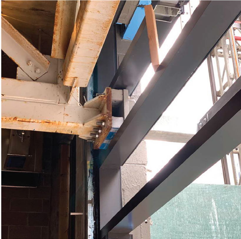
STRUCTURAL THERMAL BREAK AT CANOPY STEEL
