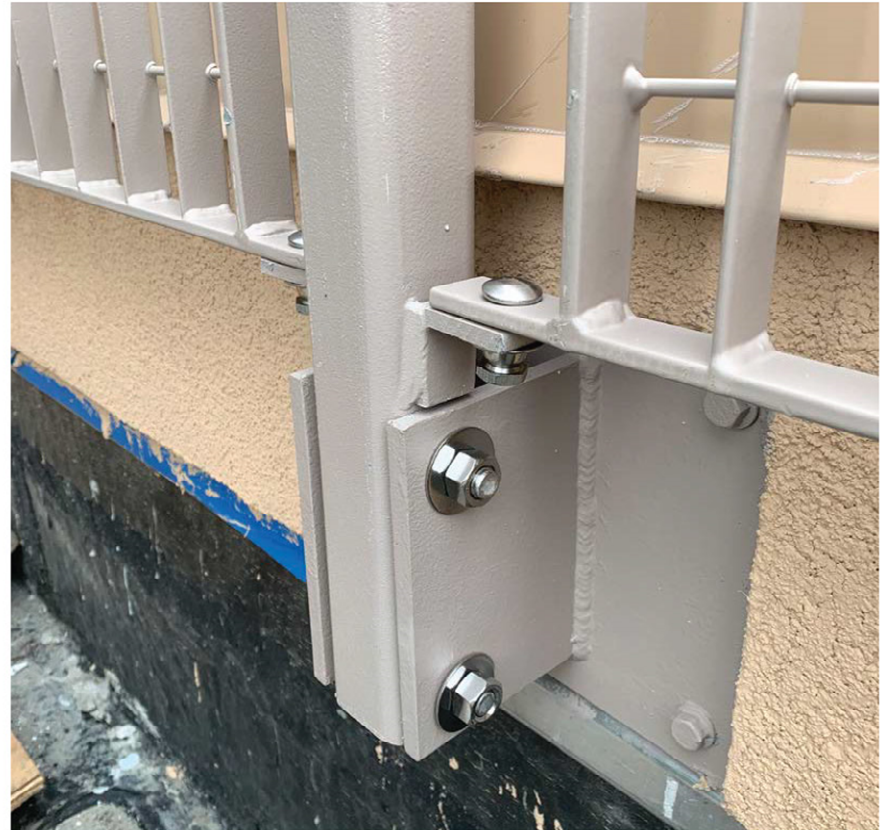
PARAPET MOUNTED RAIL @ CMU COURSES ABOVE AAC
