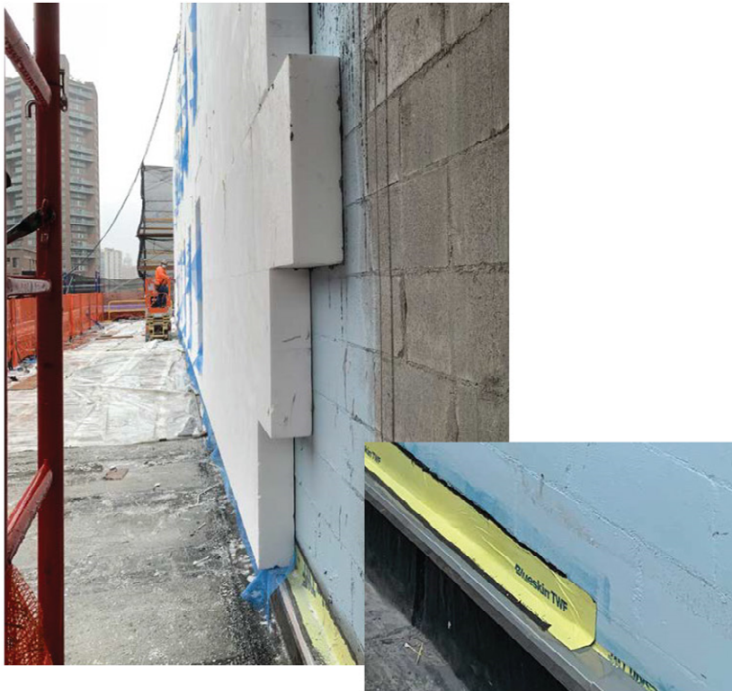
FLASHING INSTALL AT BASE OF EIFS ASSEMBLY
