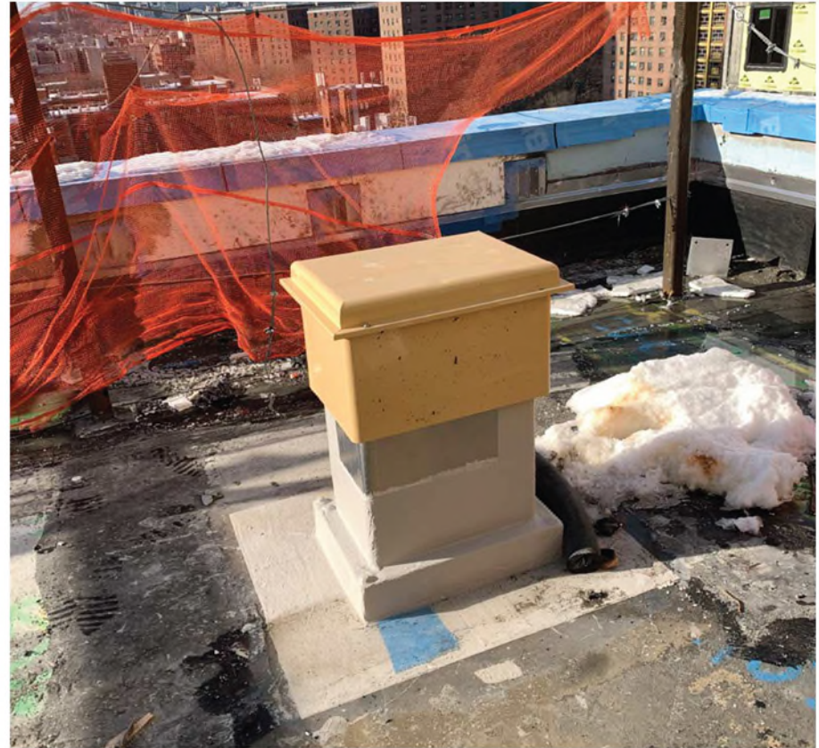
INSULATED REFRIGERANT HOUSING ON ROOF
