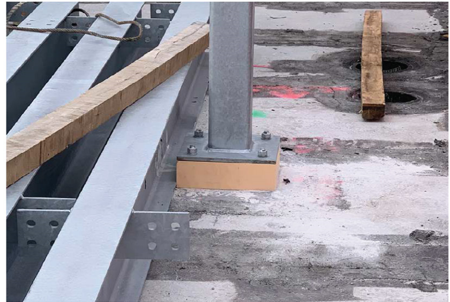
STRUCTURAL THERMAL BREAK AT PV DUNNAGE POST
