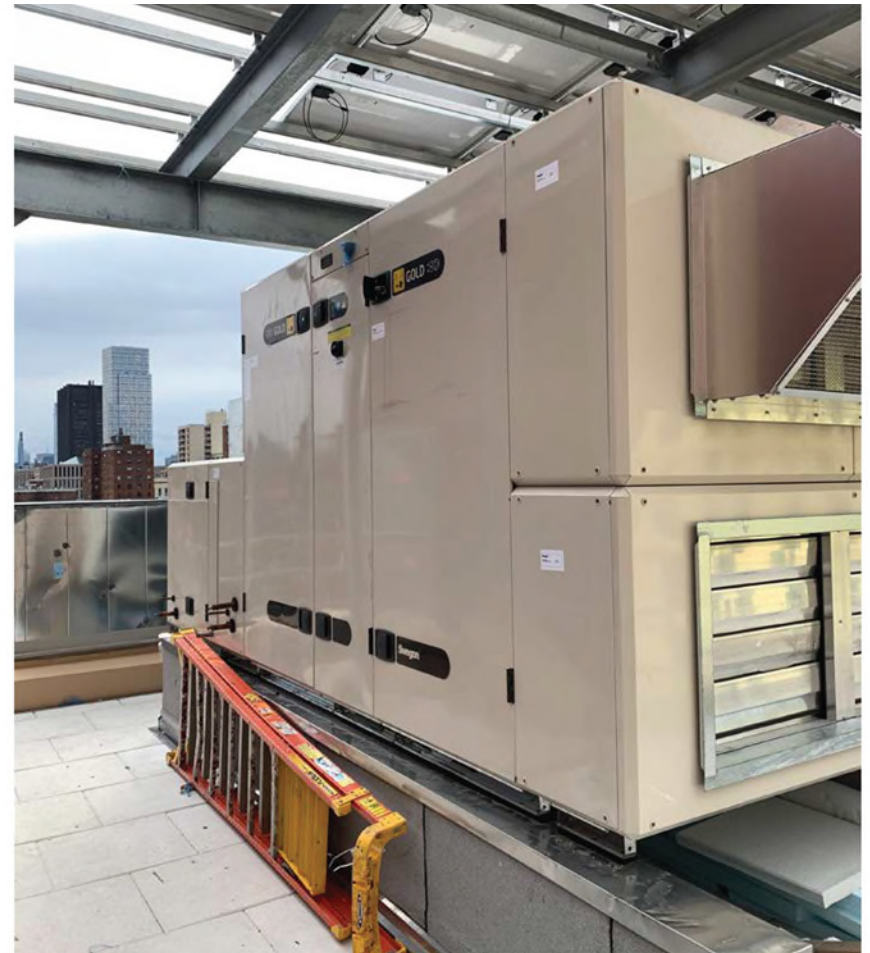
SIDE VIEW OF ERV ON THERMALLY BROKEN CURB WITH ACOUSTIC PADS
