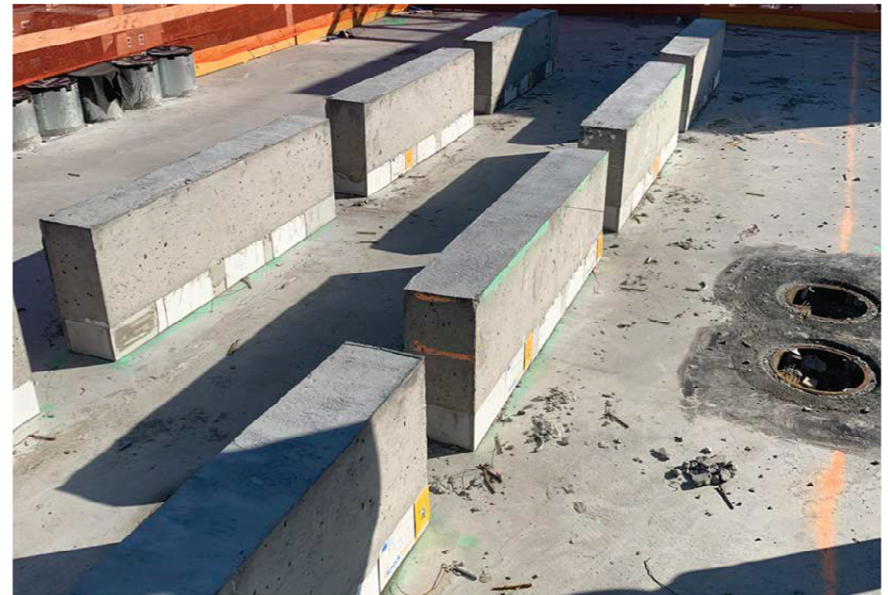
STRUCTURAL THERMAL BREAK AT GENERATOR CURBS
