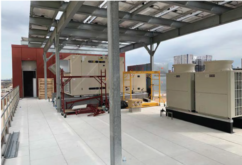
ERV WITH ASSOCIATED CONDENSERS
