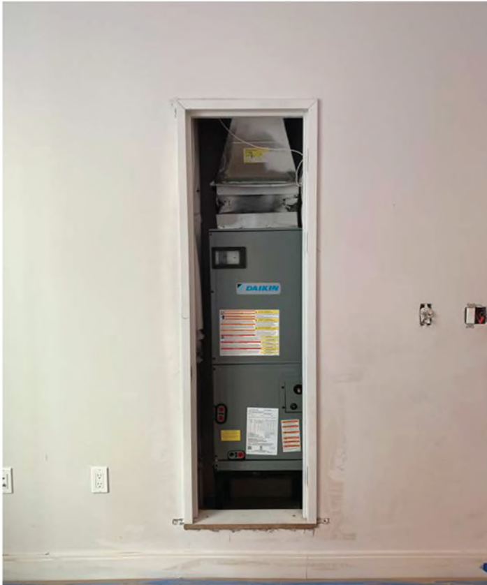
TYPICAL STANDING EVAP IN APARTMENT CLOSET
