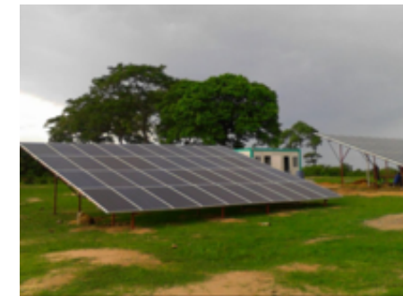
Mini-Grid system, Sinda, 30 kWp, AC, Zambia
