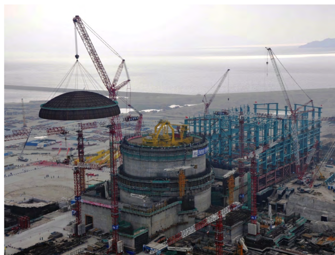
EPR under construction in Taishan, China, October 2011 (Amafrance-cn.org, CTNPJVC-EDF)
